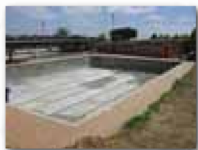
The new swimming pool under construction at Trinityhouse Randpark Ridge
